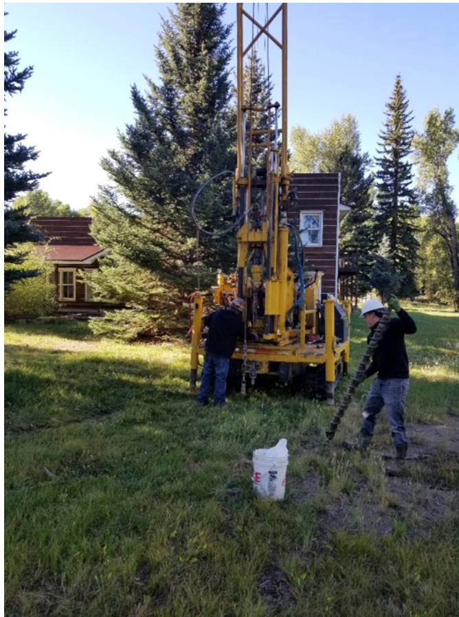
Photo 1. View looking at drilling of TH-2.
